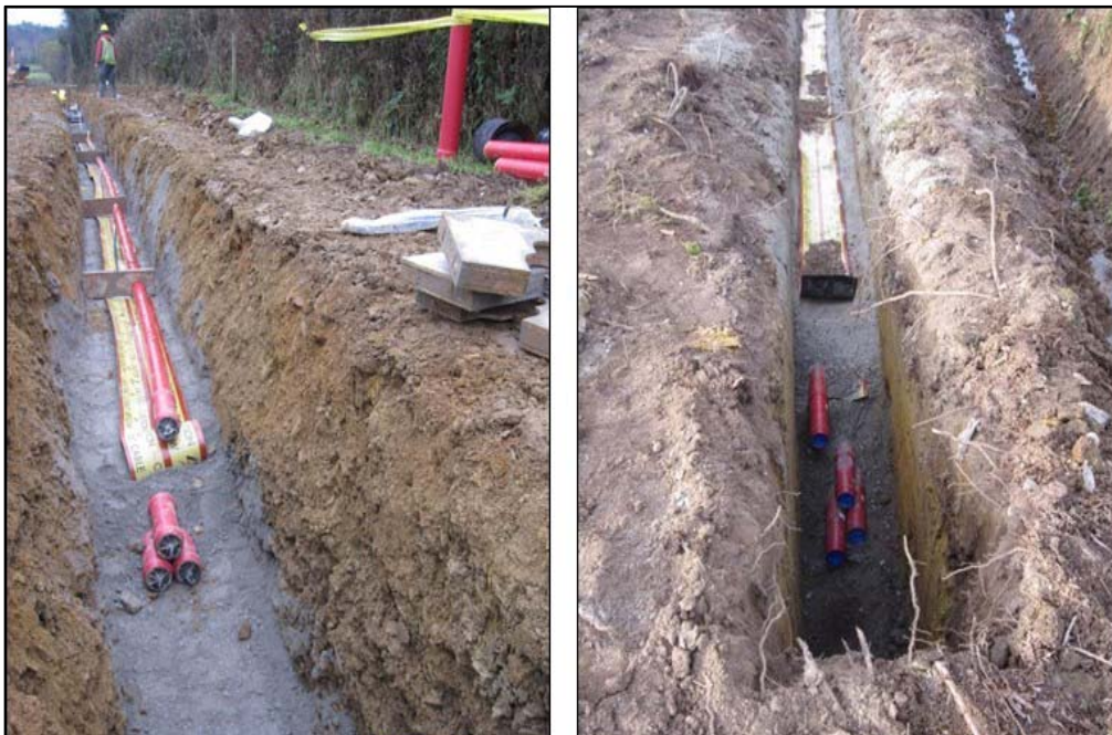
Plate 4.8 Typical Cable Trench View
