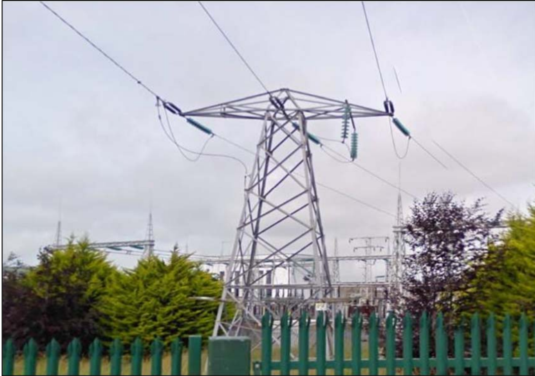
Plate 4.11 Completed End Mast Tower
