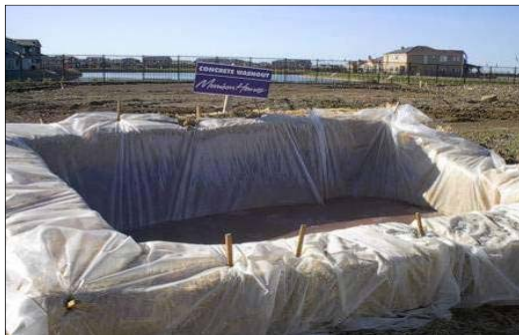
Plate 4.4 Concrete washout area
