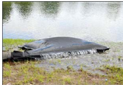
Plate 4.7 Silt bag under inspection
