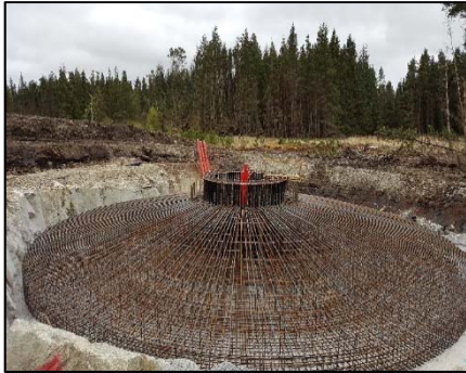
Plate 4.2 Turbine Base 'Anchor Cage'
