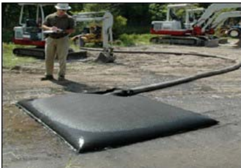
Plate 4.6 Silt Bag with water being pumped through
