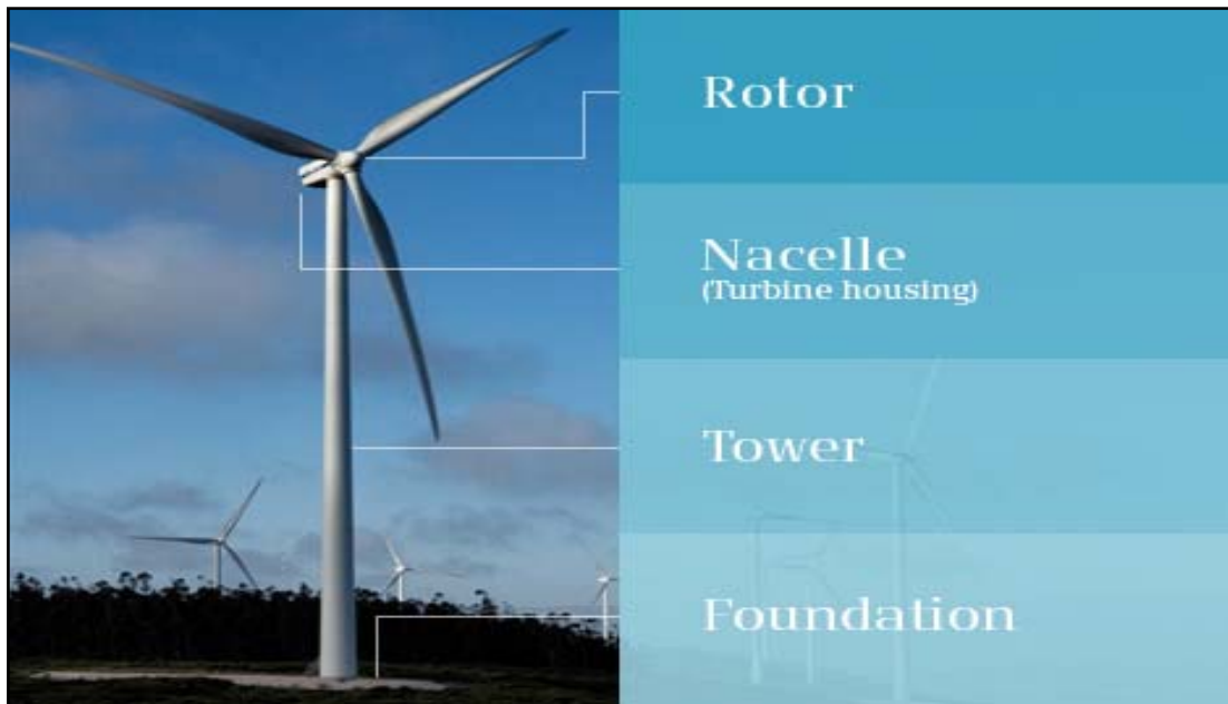
Plate 4.1 Wind Turbine Components
