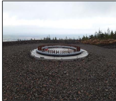
Plate 4.3 Finished Turbine Base
