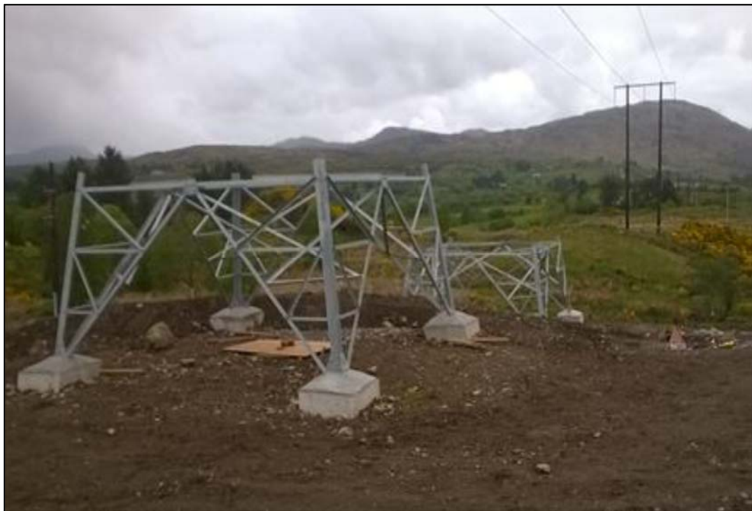
Plate 4.10 Steel lattice tower foundation complete
