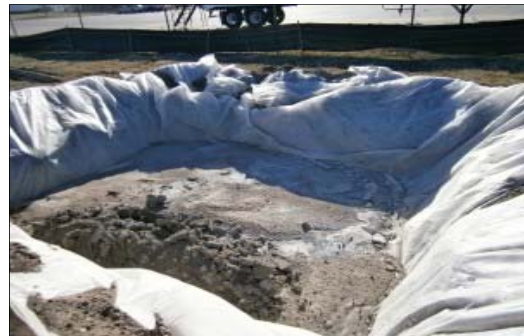
Plate 4.5 Concrete washout area
